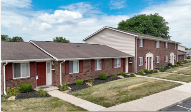
Cloverdale Heights Crawfordsville, Montgomery County
